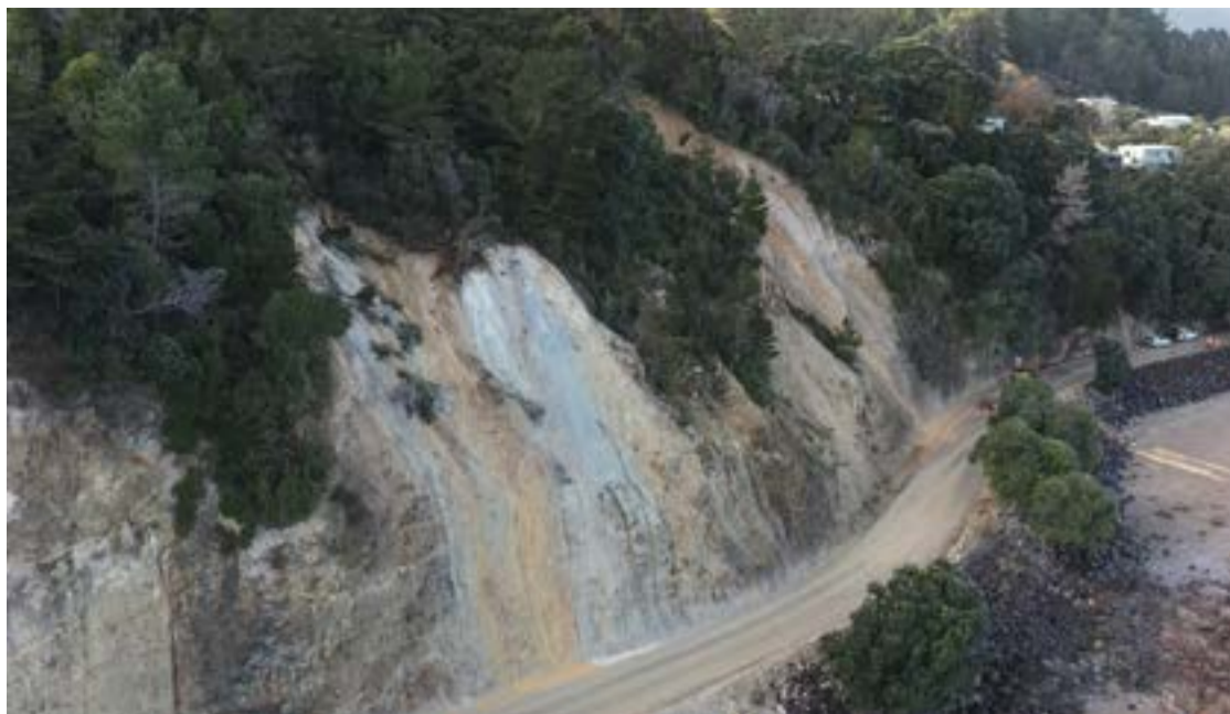
The slip site at Ruamahunga, Thames Coast.
