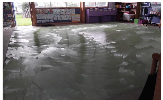
Prep work for carpet installation
